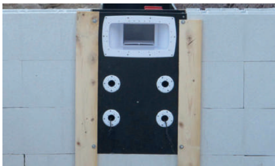
3 Install the formwork at the front and rear
