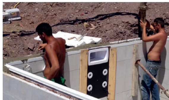
4 Cast the concrete
