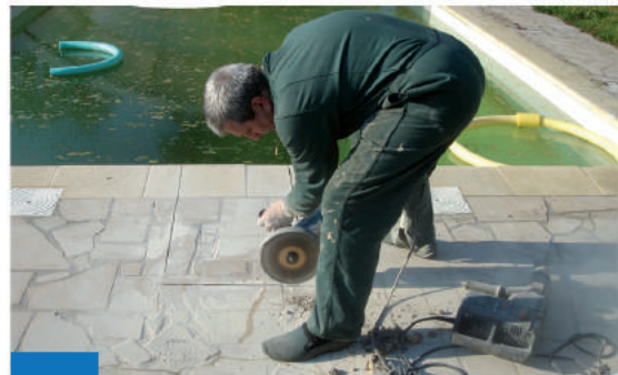
4 Cut with a diamond-saw blade
