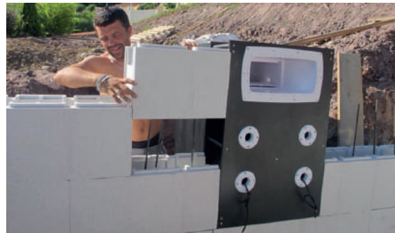
2 Build up the structure on each side of the filter wall
