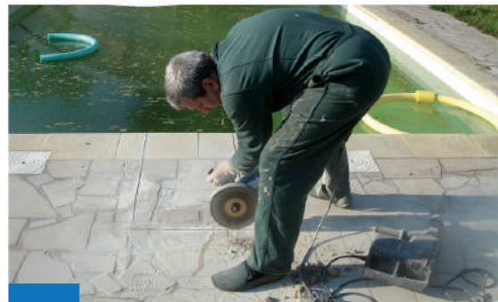
4 Cut with a diamond-saw blade
