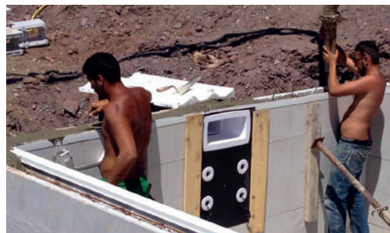
4 Cast the concrete
