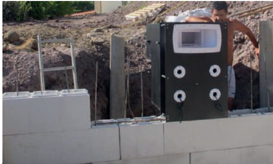
1 Place the wall on the concrete slab or on one or more rows of blocks
