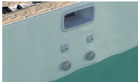
6 Seal the skimmer/nozzles/fit the spotlight
